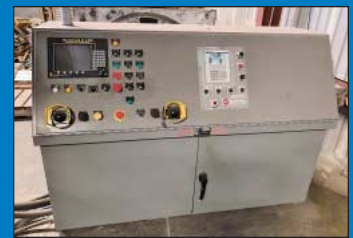
Updated Control and Electric on 400 Ton Bliss Presses
